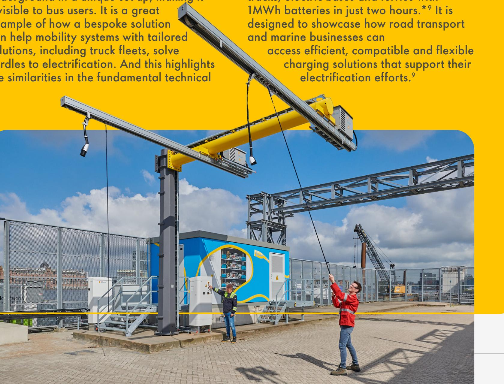
\* When charged via the Megawatt Charging System (MCS) connector, charging speeds can vary depending on factors like battery condition, ambient temperature, concurrent energy use and energy losses. Maximum continuous rating of the MCS connector is 3,000 Amps.<sup>9</sup>
